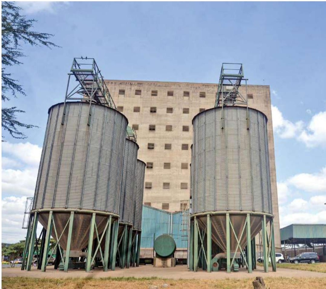
The NCPB Silos in Nairobi. Picture | File
